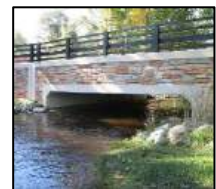
Figure 4: Three-sided box bridge
