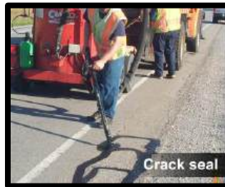
Figure 6: Examples of capital preventive maintenance
