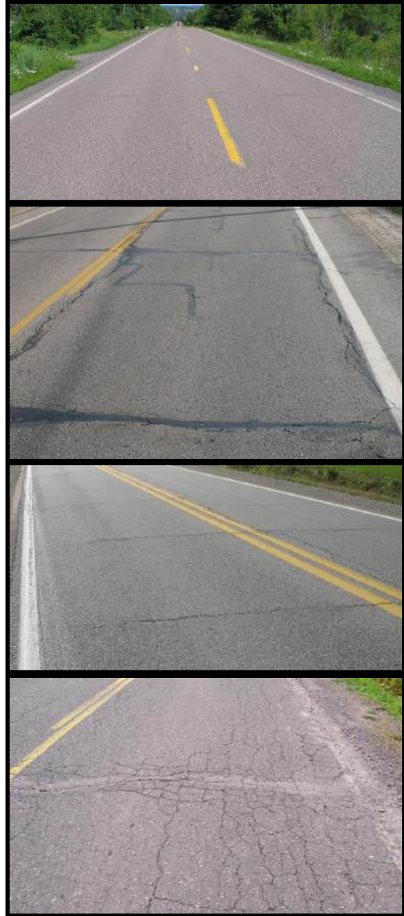
Figure 3: Top image – PASER 8 (Good). Second image – PASER 5 (Fair). Third image – PASER 6 (Fair). Bottom image – PASER 2 (Poor).
