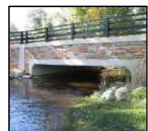
Figure 4: Three-sided box bridge
