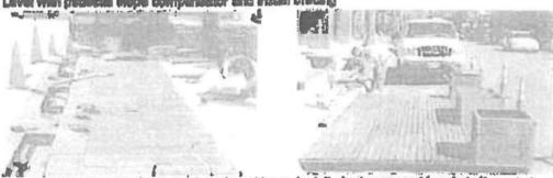
Completed bracing, Anchor to outb and road base. Install planter support brack
