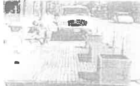
Completed bracing. Anchor to curb and road base. Install planter support brackets if needed.
