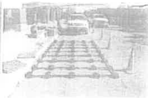
Set pedestals roughly 2 feet apart
