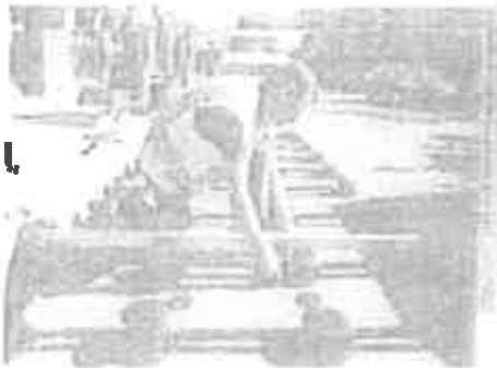
Level with pedestal slope compensator and install bracing
